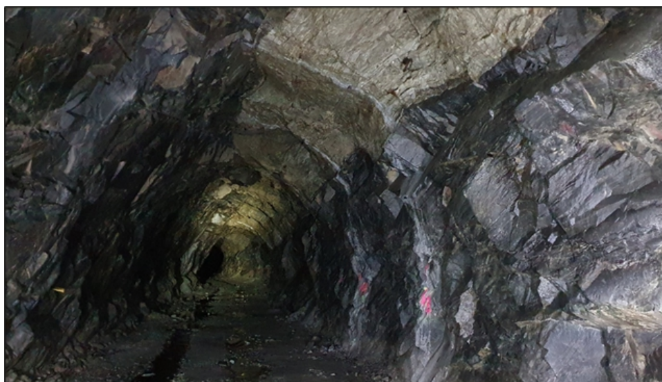
Figure 9-10: Pegmatite exposure in the roof of an exploration drift Source: CSA Global
