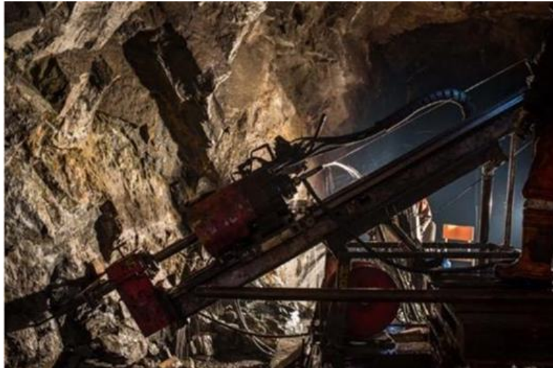
Figure 7-2: A Sandvik DE130 rig drilling drillhole number P15-22 Source: European Lithium/DRA
