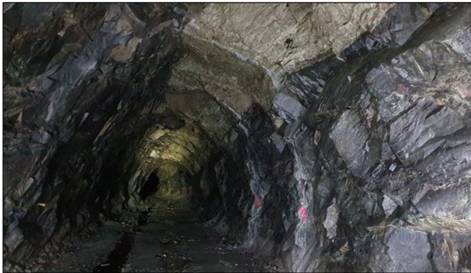
Figure 9-10: Pegmatite exposure in the roof of an exploration drift Source: CSA Global
