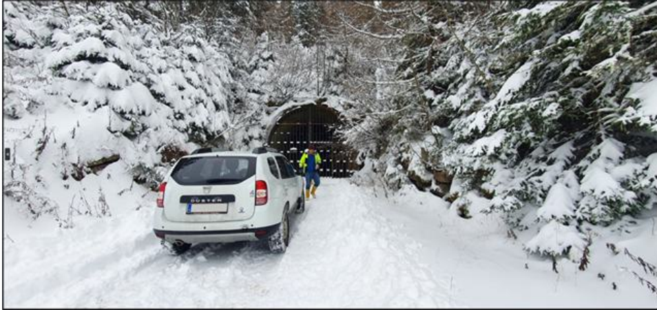
Figure 9-8: Portal entrance at the Wolfsberg underground mine Source: CSA Global
